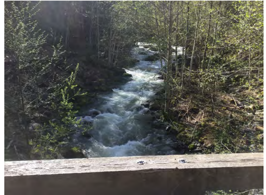
Looking upstream from deck
