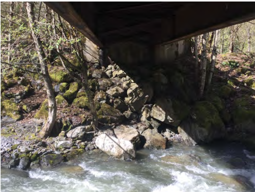
Left Bank Abutment when facing downstream
