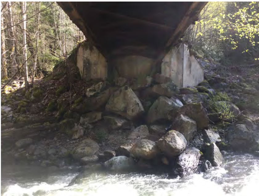
Right Bank Abutment when facing downstream
